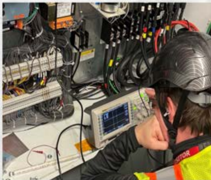
Field work/installation; image courtesy of Delaware Elevator
