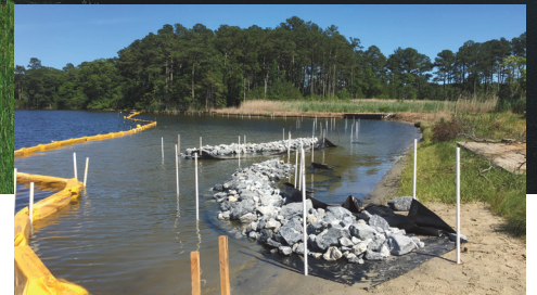
The installation of the rock sill. The area behind these rocks was filled with sand and planted with native grasses
