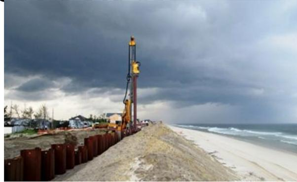
BURIED FLOODWALL / STRUCTURAL DUNE
