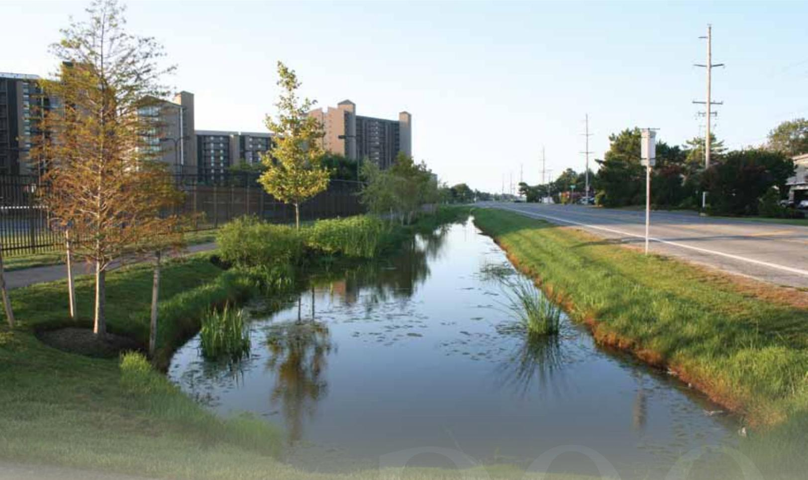
*Once a ditch to convey stormwater runoff, this area was widened, deepened, and planted with native vegetation to detain runoff so that less sediment, nitrogen, and phosphorus enters Little Assawoman Bay. Photo credit: Chris Bason*
